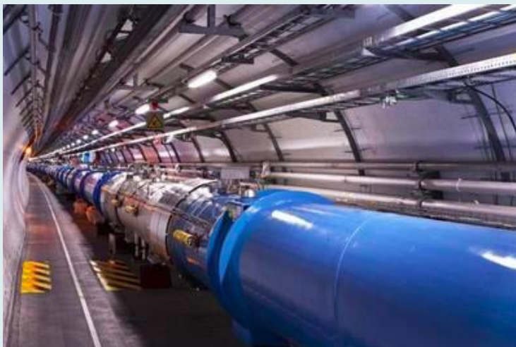
Picture 3 CERN tunnel https://www.flickr.com/photos/miniprince/10007299826/
